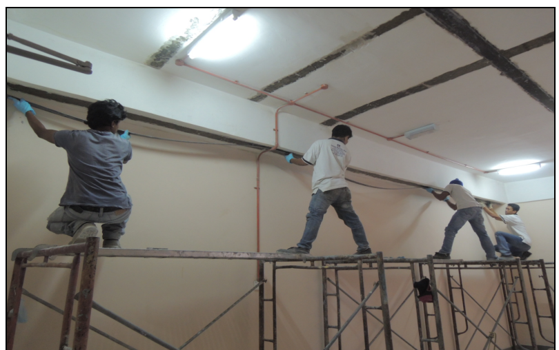
Build Strip HM 1014, apply on Beam
